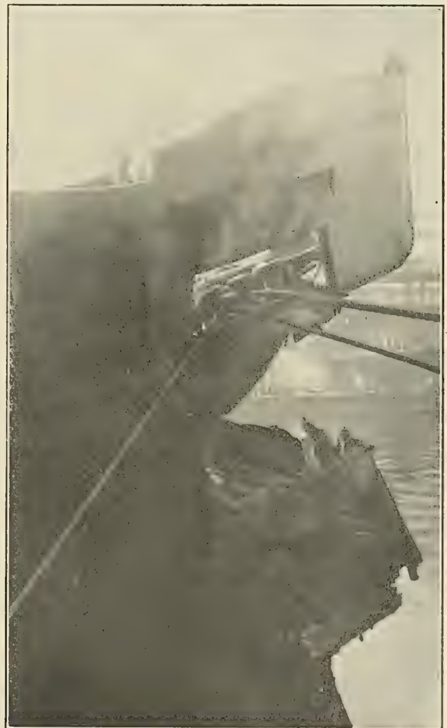
SIDE VIEW, SHOWING DAMAGE TO BOW OF HURONA.
